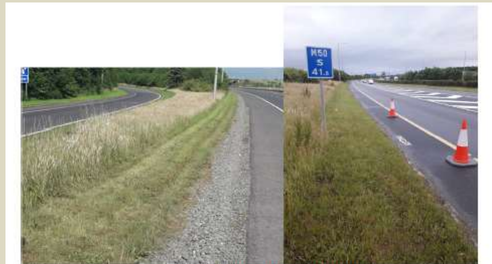
2m verge and interchange grass cut
